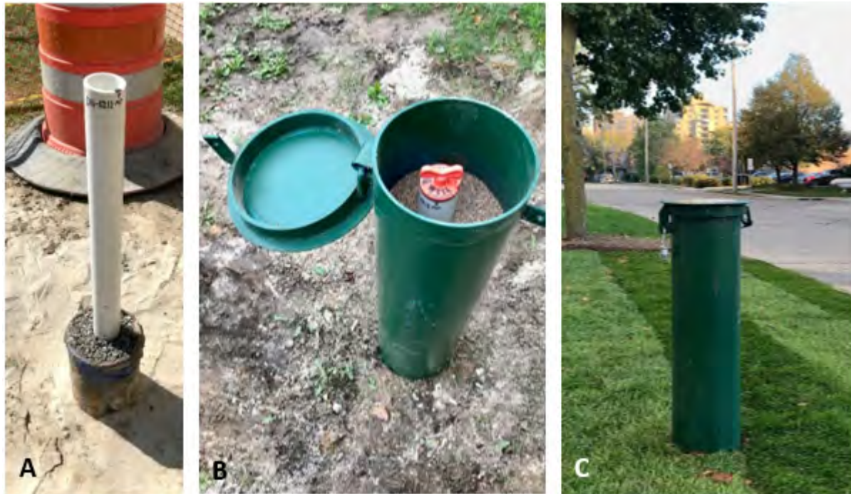
Figure 27. Well DN-6212 (replacement for well DN-1297). Panel A, completed will DN-6212 with several inches of above-grade steel casing surrounding 2-in.-diameter PVC casing completed with a 5-ft-long well screen connected to the sandstone bedrock aquifer at the bottom. Panel B, locking steel protective well head cover installed around well DN-6212. Panel C, completed well DN-6212 west of the Kohl center after landscaping completed at the site.
