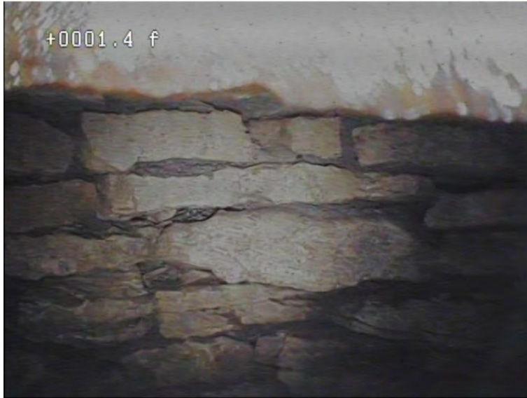
Figure 72. Video screenshot from VE-08 borehole video collected on November 17, 2021; footage on image is in depth below top of casing (also the land surface datum) as recorded by the video logging equipment. Side-hole view of the bottom of the 4-in.-diameter casing and original rock-lined wall of the hand-dug well.
