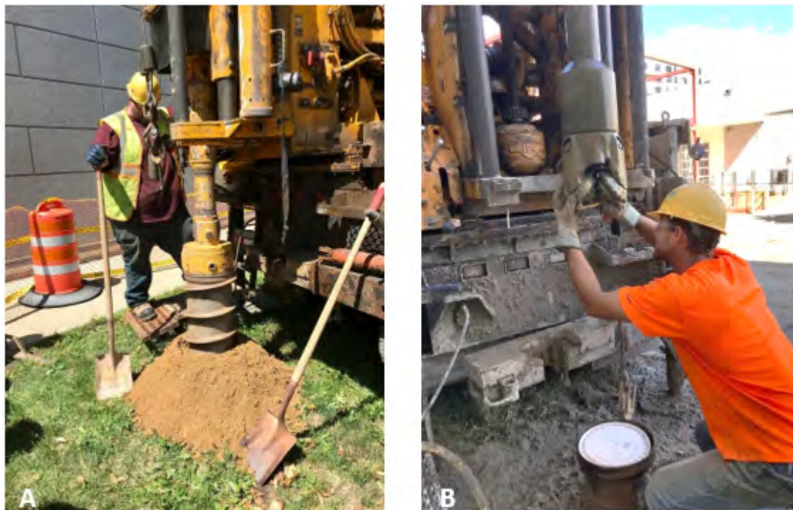
Figure 25. Soils and Engineering Services, Inc. drilling well DN-6212 (replacement for well DN-1297) on the east side of the Kohl Center building on the University of Wisconsin-Madison campus. Panel A, hollow stem auger being used to bore through the unconsolidated material overlying bedrock. Note the eastern wall of the Kohl Center behind the driller. Panel B, 10-in.-diameter air rotary drill bit used to bore through bedrock from approximately 80 to 88 ft blsd. White cap in steel pipe located beneath the drill bit, is the DN-6212 borehole.
