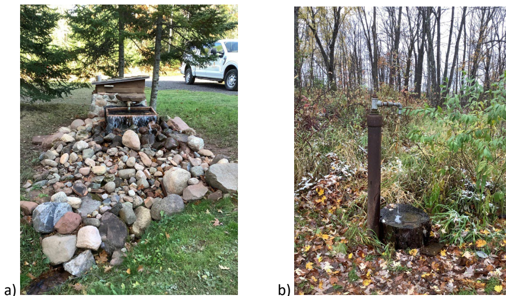
Figure 11. Examples of erosion-control measures near the point of discharge of a flowing well. a) Boulders and cobbles (BA-FW-37), b) Tree stump (BA-FW-04).
