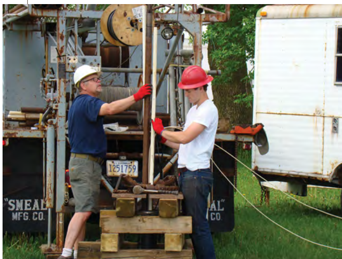
Placing a pump discharge pipe for hydraulic tests.
