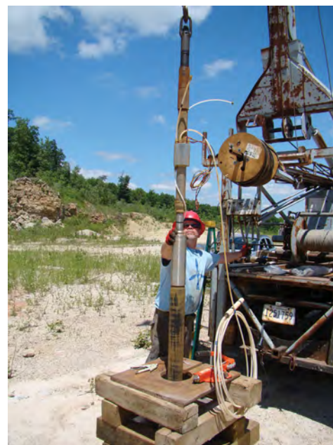
Installing packer and pump into a well for hydraulic tests.
