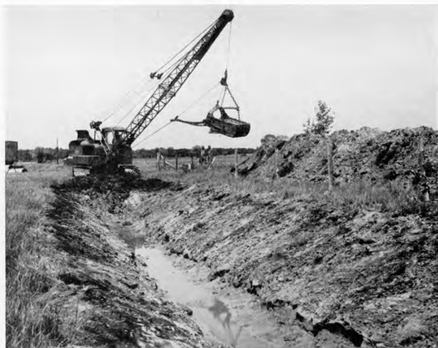
Figure 36. Creating new cropland by land drainage.
